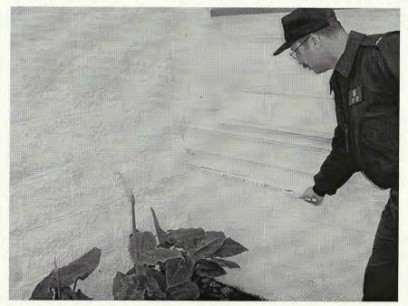
Photo #4 shows the exterior of the front porch with a settlement crack.
